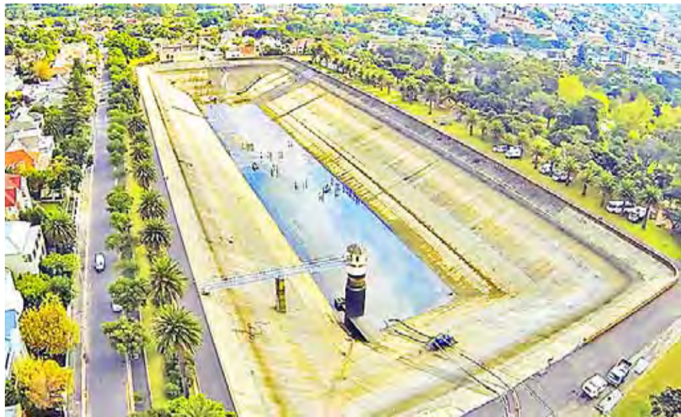
The Molteno Reservoir in Cape Town.
