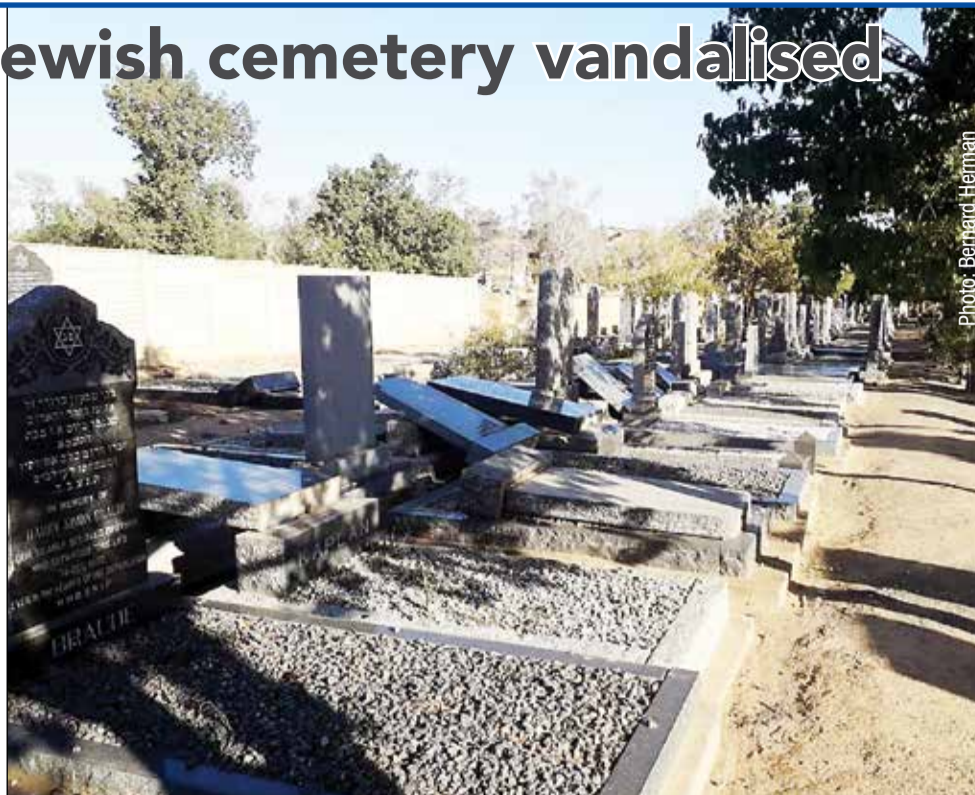
Some of the vandalised graves in the Oudtshoorn Jewish cemetery
