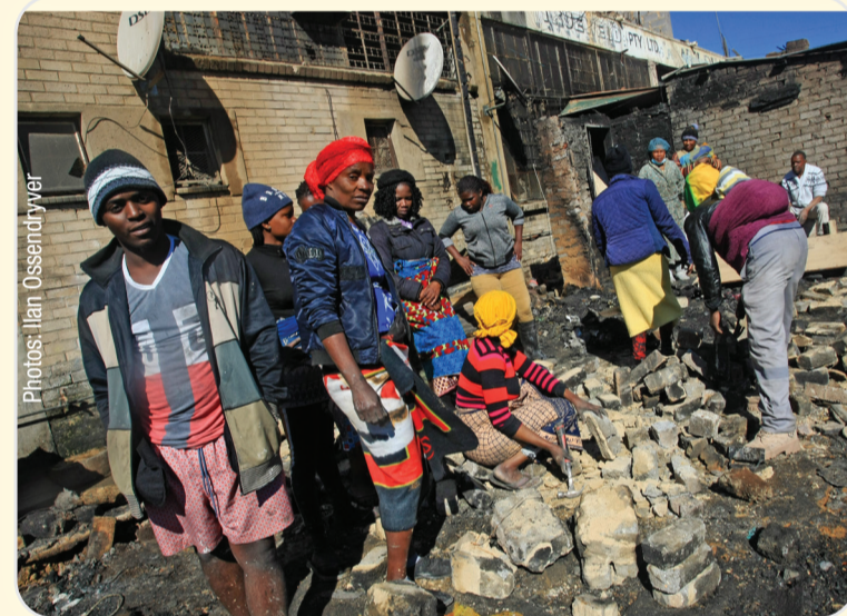
Alexandra residents rebuilding five houses that were destroyed during the rioting
